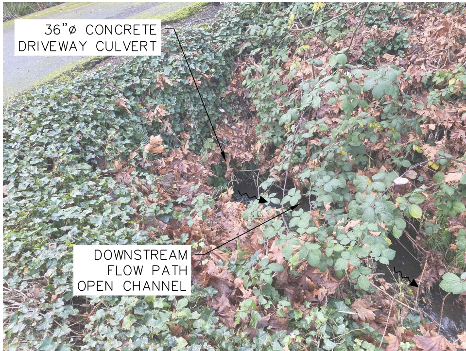
MERCER ISLAND STORM DRAIN CHANNEL WEST OF 76TH AVE SE
