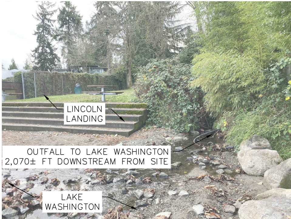
MERCER ISLAND STORM DRAIN CHANNEL OUTFALL TO AT LINCOLN LANDING
