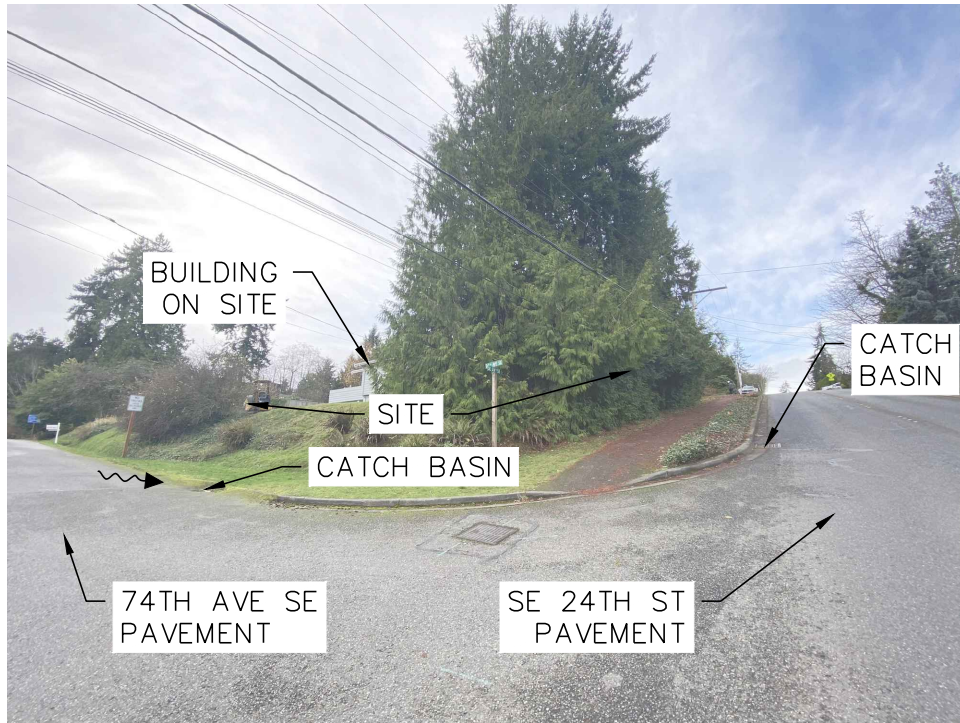
CORNER OF 74TH AVE SE AND SE 24TH ST LOOKING SOUTHWEST AT SITE
